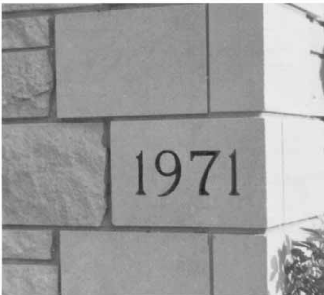
Front-facing quoins are prime locations for date stones or street addresses. Most suppliers can arrange lettering, numbers and other inscriptions.
